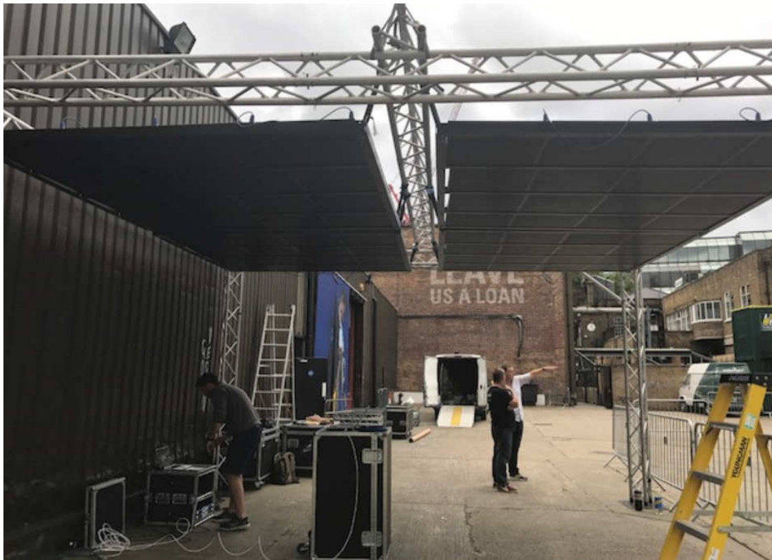
Photo 1 : Zone Array dancefloor speaker system providing the sound source
